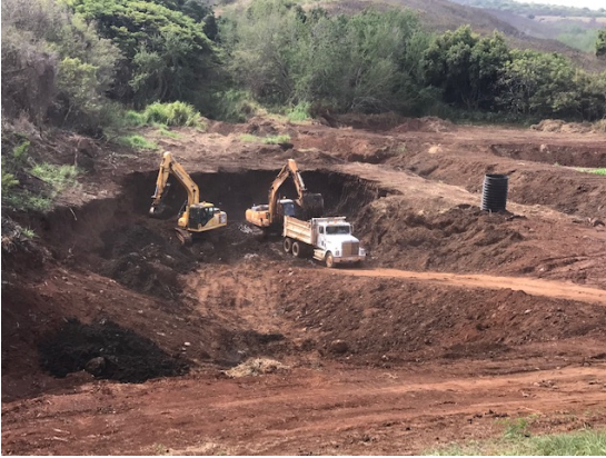
Clearing out twenty years of accumulated sediment at Kahana Nui basin, West Maui to restore capacity. Credit: West Maui R2R
